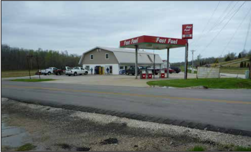
Photo 21: Potential hazardous materials concern site (UST record) at Weber Store/BP 455 Fast Fuel gas station; KY144 roadway right-of-way in foreground; facing northwest.
