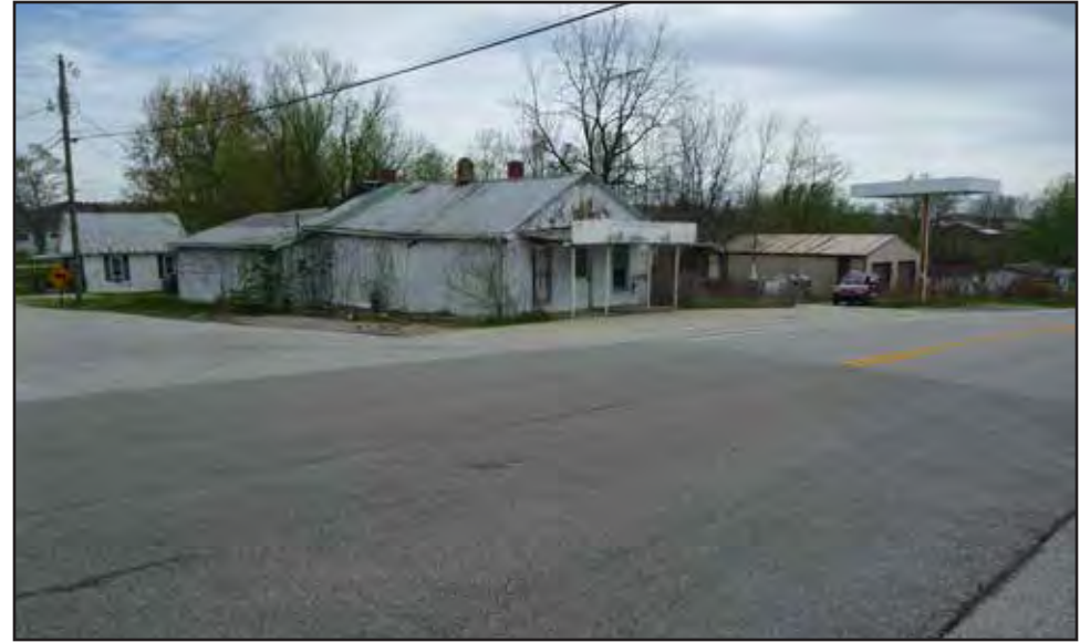
Photo 22: Potential hazardous materials concern site (UST record) at vacant Roseville General Store (former gas station); existing roadway right-of-way at intersection of KY69 and Pellville Road (foreground); facing southeast.
