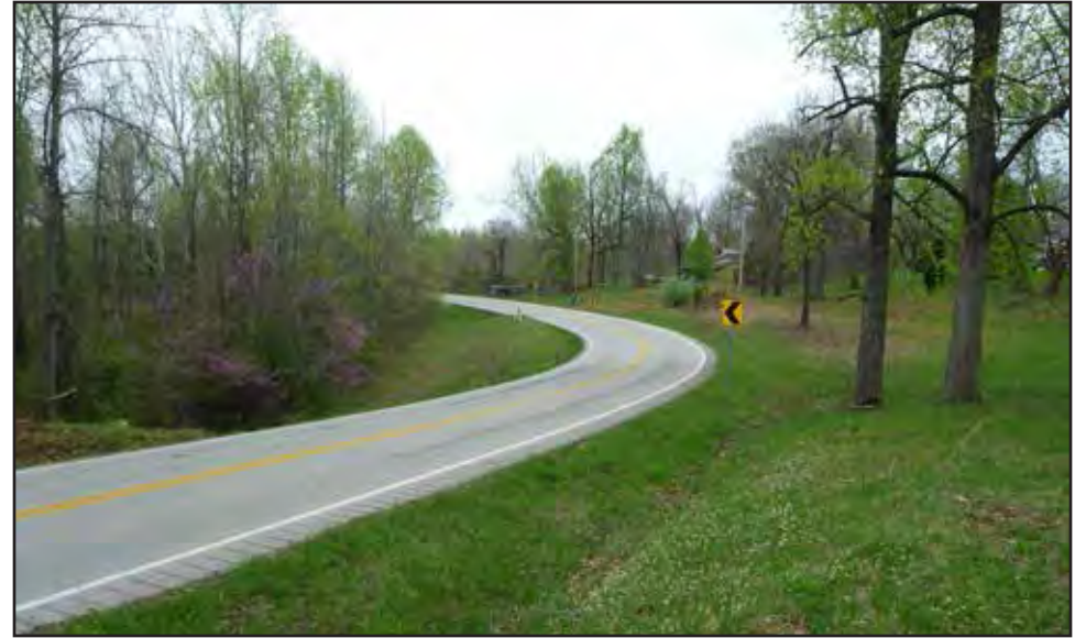
Photo 46: General view of existing roadway right-of-way; sharp curve on KY69; facing north.
