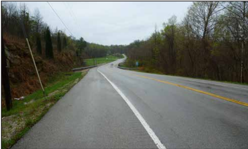
Photo 43: General view of existing roadway right-of-way; KY69; facing southwest.
