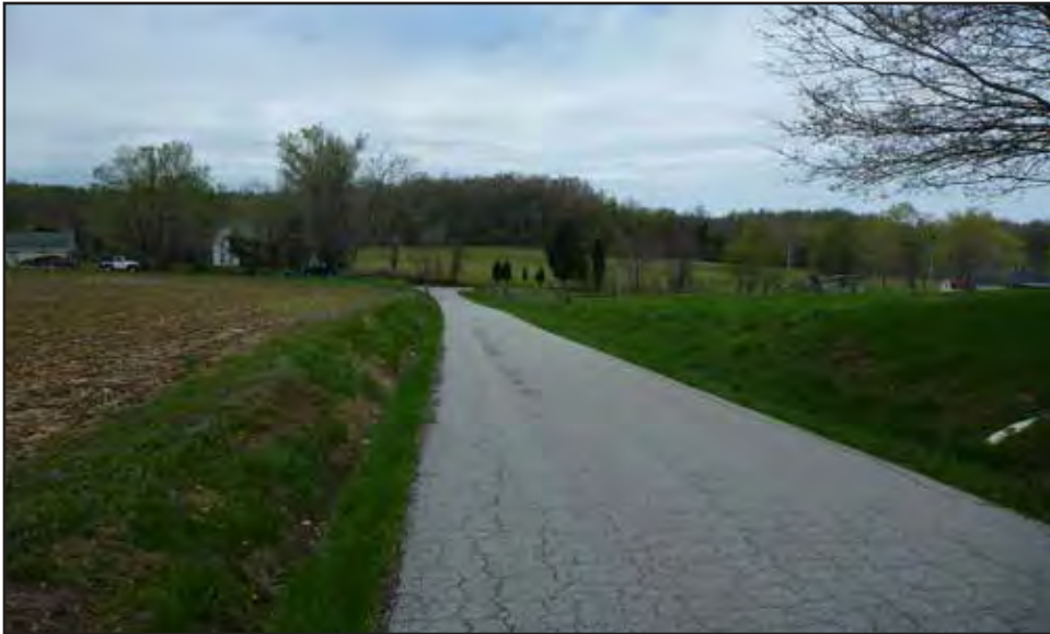
Photo 47: General view of existing roadway right-of-way; Luke Mercer Road; facing northwest.
