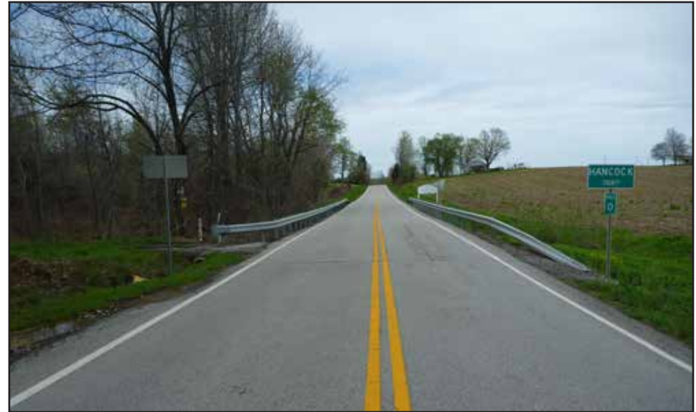
Photo 48: General view of existing roadway right-of-way; KY69 at the Hancock County line; facing northeast.
