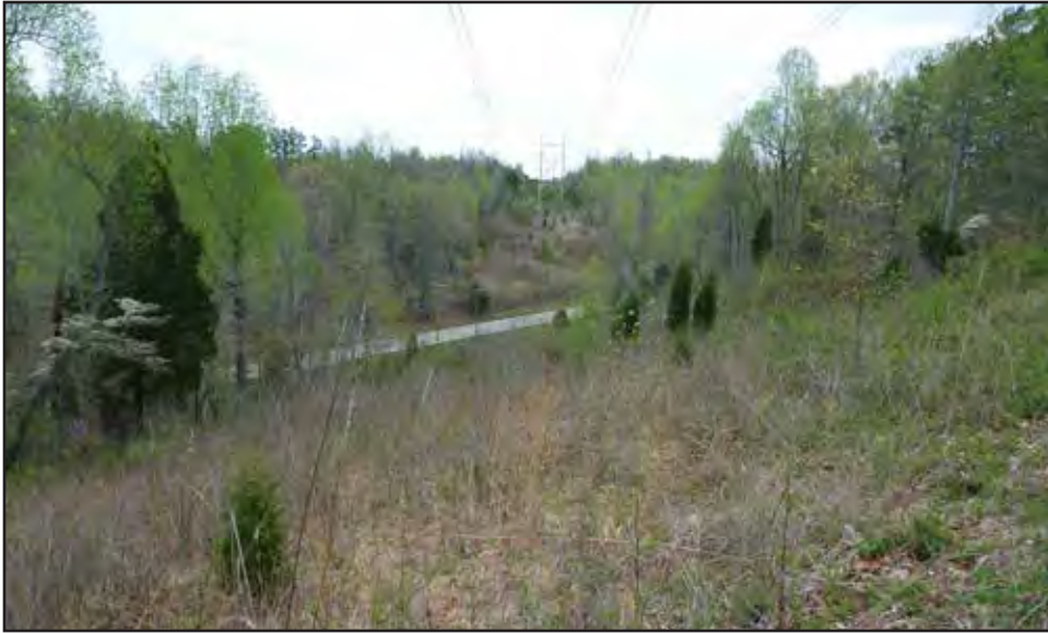
Photo 29: Existing utility crossing; electrical transmission line; surrounded by upland forest habitat; facing east.
