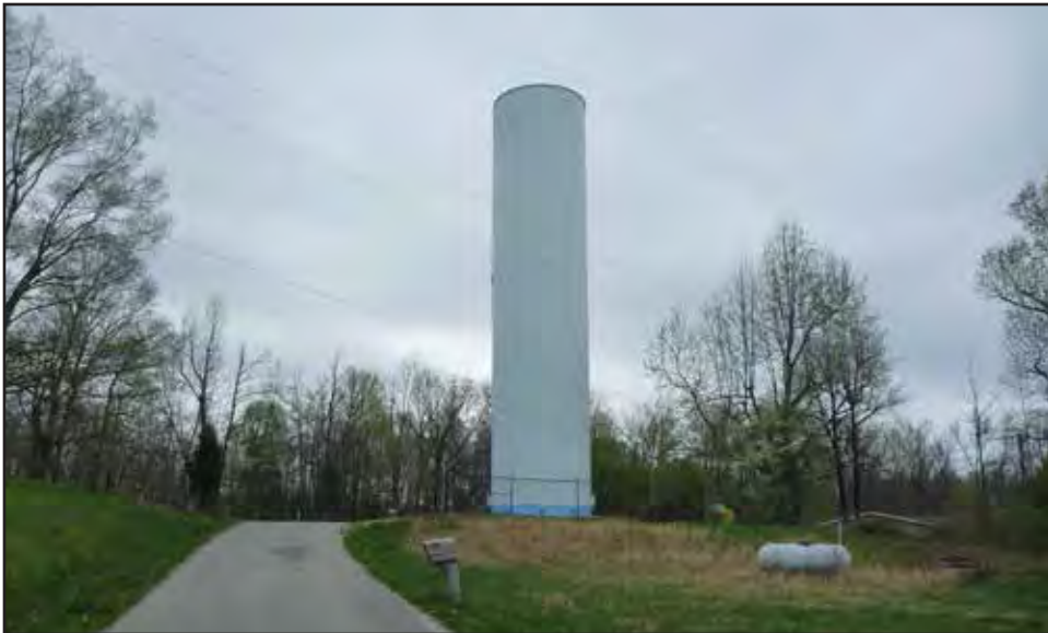
Photo 31: Existing utility; water tower off Water Tower Loop road; facing south.
