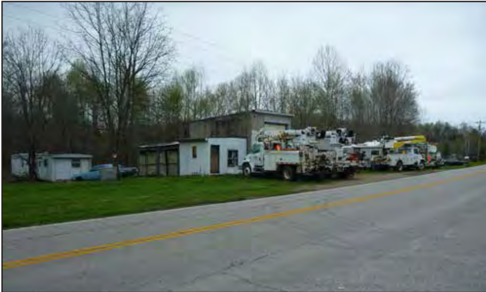
Photo 27: Potential hazardous materials concern site; possible former garage along KY69; facing northwest.
