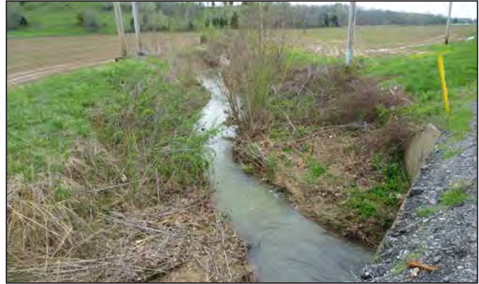
Photo 6: Unnamed Tributary to Horse Fork, USGS-perennial, open riparian corridor; looking downstream from KY69 culvert; agricultural land use (row crop) in background; facing northwest.
